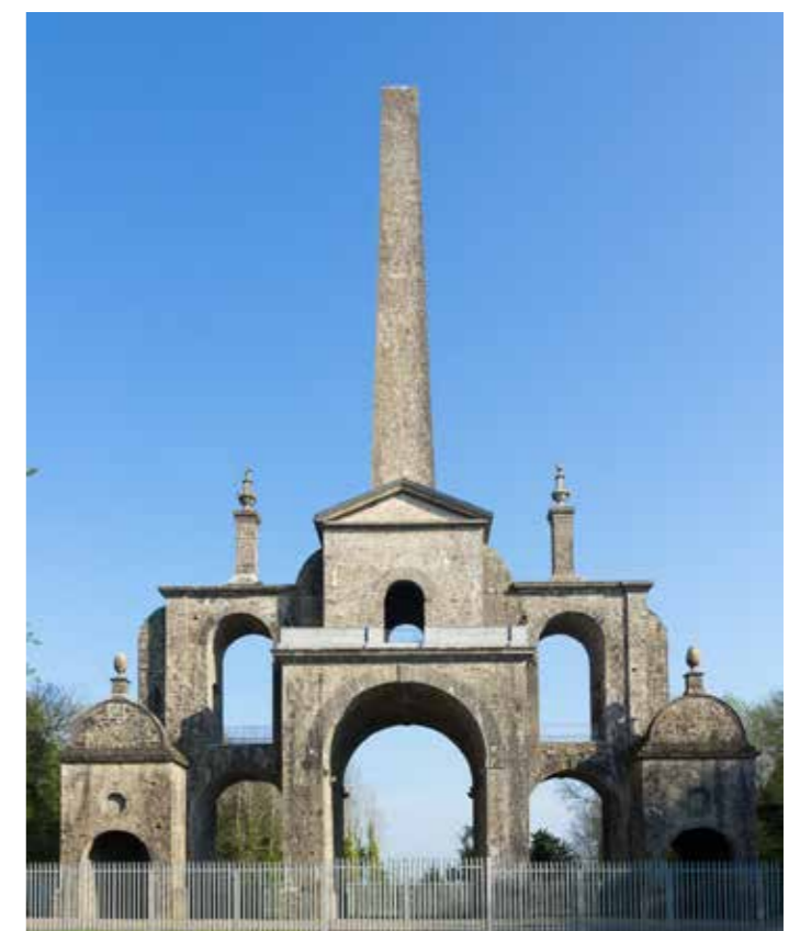
Conolly's Folly, as it is today with a metal fence surrounding it.
