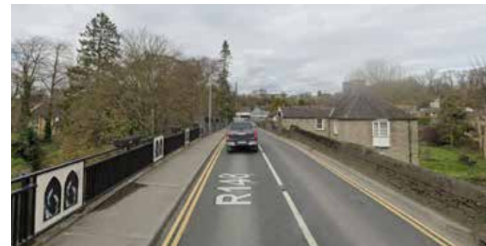
Google Street View- Salmon Leap Bridge with narrow carriageway and Pavement to one side only.
