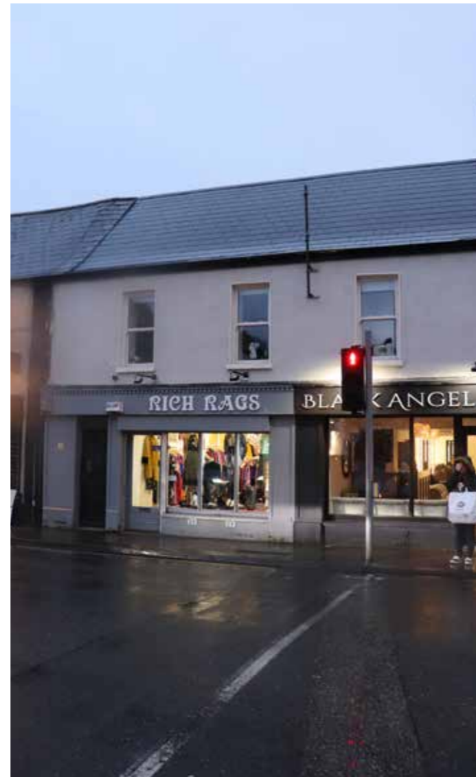
Typical Main Street shop fronts
