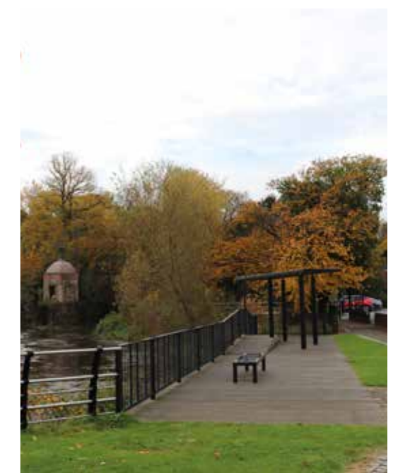
Existing Pavilion on Heritage Trail
