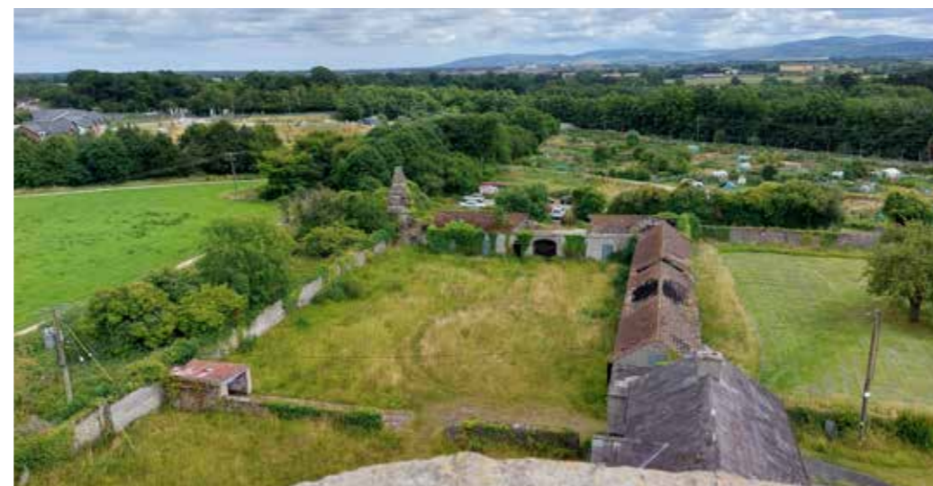
View from top of barn (looking east)
